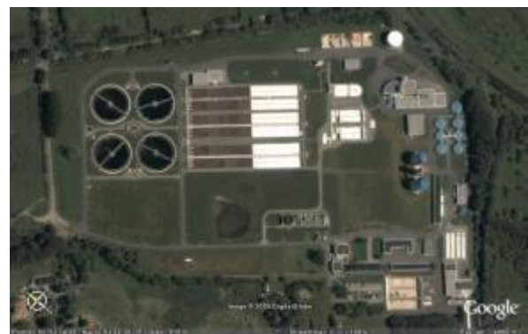
Aerial picture of the WWTP Chemnitz (source: google)
